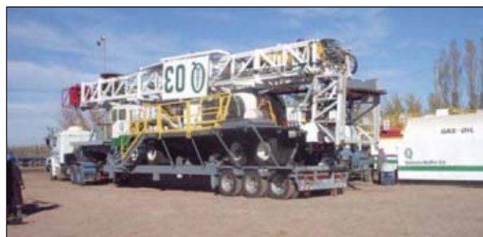
Quintana WellPro’s Rig 3, a National Oil Well 400 model, was preparing to drill for Petrolifera Petroleum in the Rinconada Block, Neuquen basin (photo from Petrolifera Petroleum Ltd., Fig. 3).
