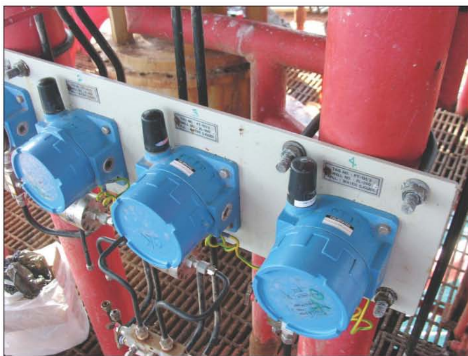
Wireless sensors are less bulky than traditional SCADA installations (Fig. 4).
