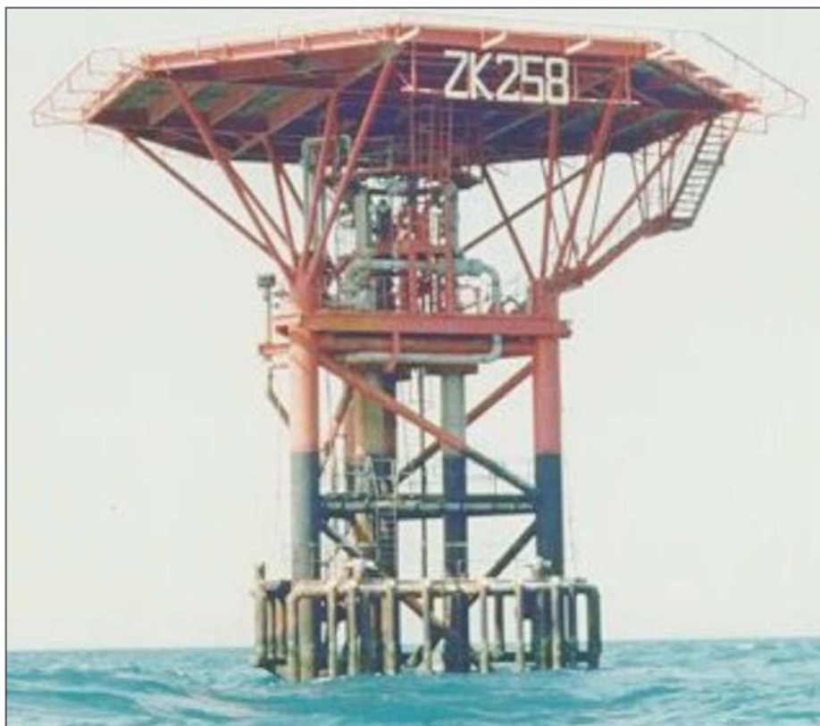
Lower Zakum field off Abu Dhabi has more than 110 water-injection wells on about 26 platforms (Fig. 1).
